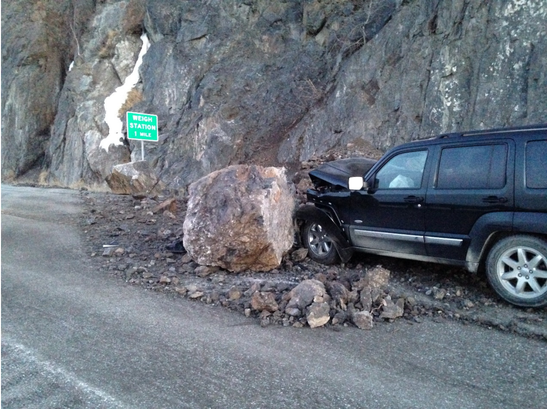
Exhibit 6. February 2015 rock slope failure close call on the Seward Highway
