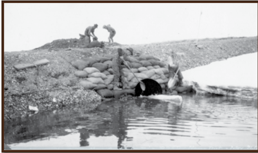
Men working on an embankment and culvert near Nome, filling sandbags to protect the road.
