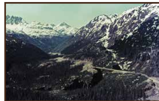
Klondike Highway, looking back toward Skagway, May 1977.
