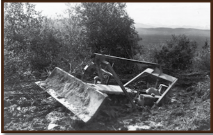
Road construction equipment in deep mud.
