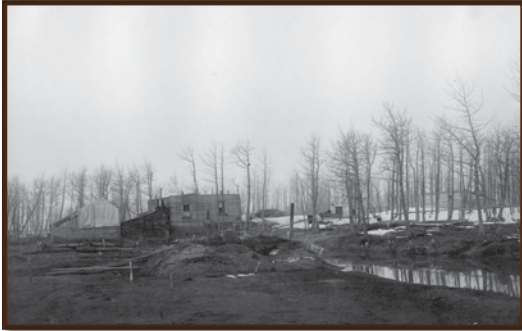
Buildings at Pilgrim Hot Springs, Alaska.
