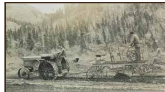
An Alaska Road Commission construction crew grading a road with a case tractor.
