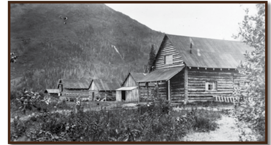
A camp of the Canyon Creek Development Company at Mile 29 of the Seward Highway.
