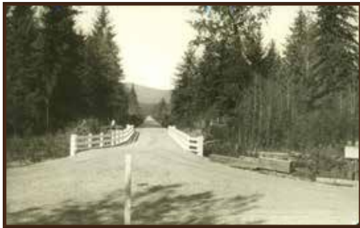
A short bridge along the Glacier Highway near Juneau, built by the Bureau of Public Roads. Alaska State Library, George A. Parks Photo Collection ASL-P240-235
