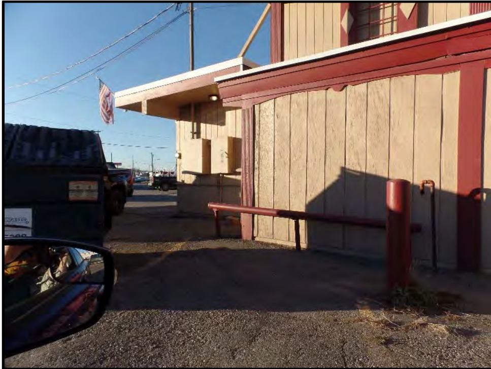
Photo 7: View of the buried heating oil tank located on Parcel 4.
