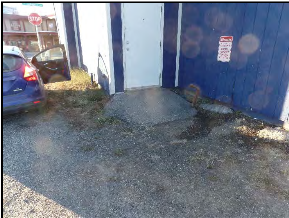
Photo 8: View of the buried heating oil tank located on Parcel 11.
